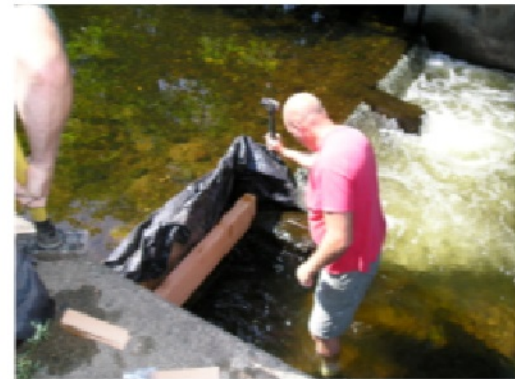
Joe Hall, from Jacobson Landscaping, installs the new stop log.
