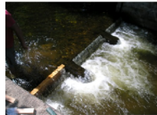
The stop log in it's new home.
