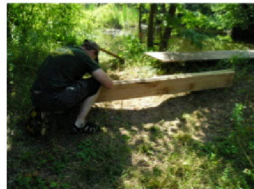
Joel Jacobson, from Jacobson Landscaping, carefully measures the cut line for the new stop log.
